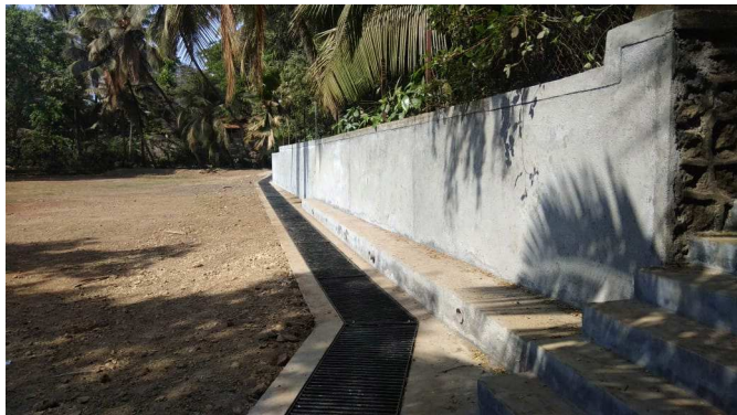
A supporting wall and a diversion for rainwaters have been completed.
