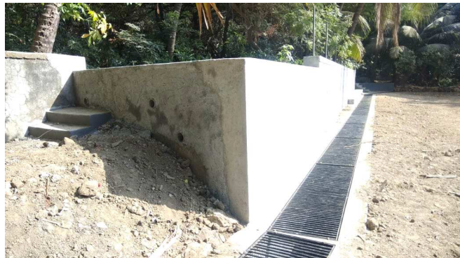
A supporting wall and a diversion for rainwaters have been completed.
